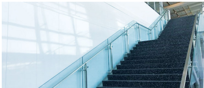
450' of Stacked Walls With Varying Heights San Diego International Airport | San Diego, CA
