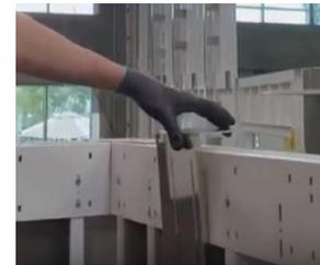
2. Attach each sliding bracket loosely to the back of the top rail of a modular system, placing each one near the ends of the top trim cap.
