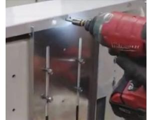
6. Once the sliding brackets are secured to the adjustable top trim cap, slide the trim cap upward to the desired height, closing off the gap between the modular walls and the ceiling.
